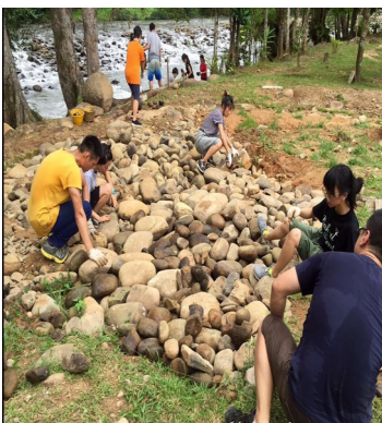
Laying a foundation for a building
